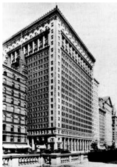
Burnham, People's Gas building, 1910
